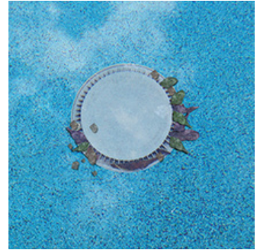
Typical pool drain with debris unable to exit pool
